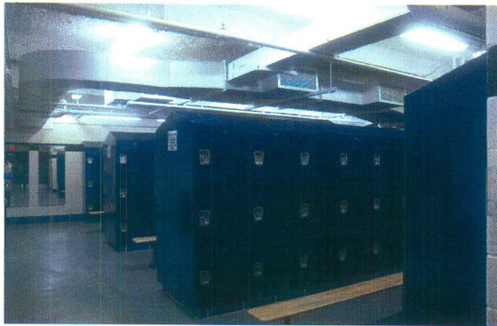
New Trier High School - Winnetka Campus Locker Room Renovation
