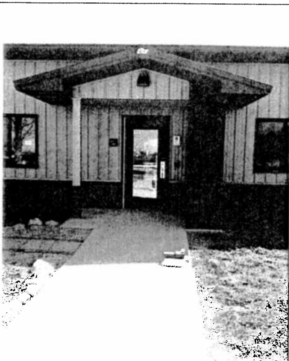
View outside Subject Building. Location for Sample 21137430.
